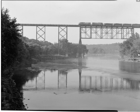
River Span across the Des Moines River including the unique Bents on either side.
