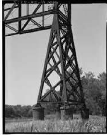
River Span across the Des Moines River including the unique Bents on either side.
